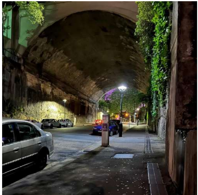
Figure 16: Argyle Cut underpass on Argyle Street
