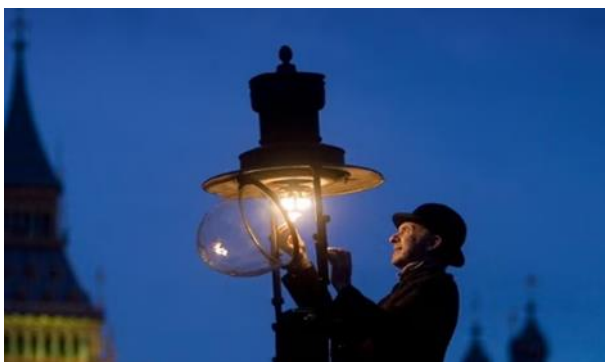
Figure 5.7 Street light maintenance, The Times
