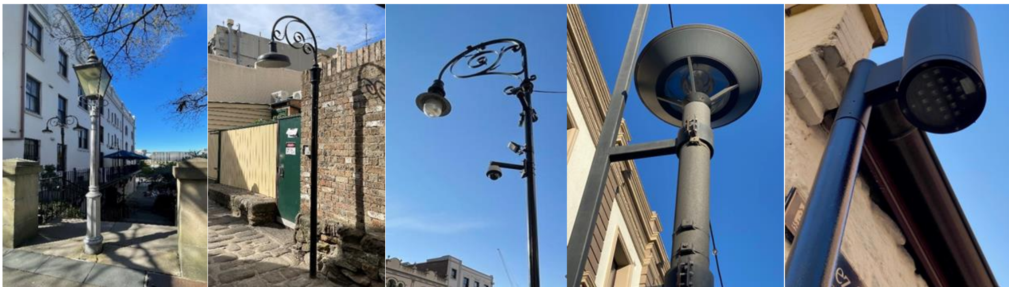
Figure 3.8 Selection of existing streetlights
