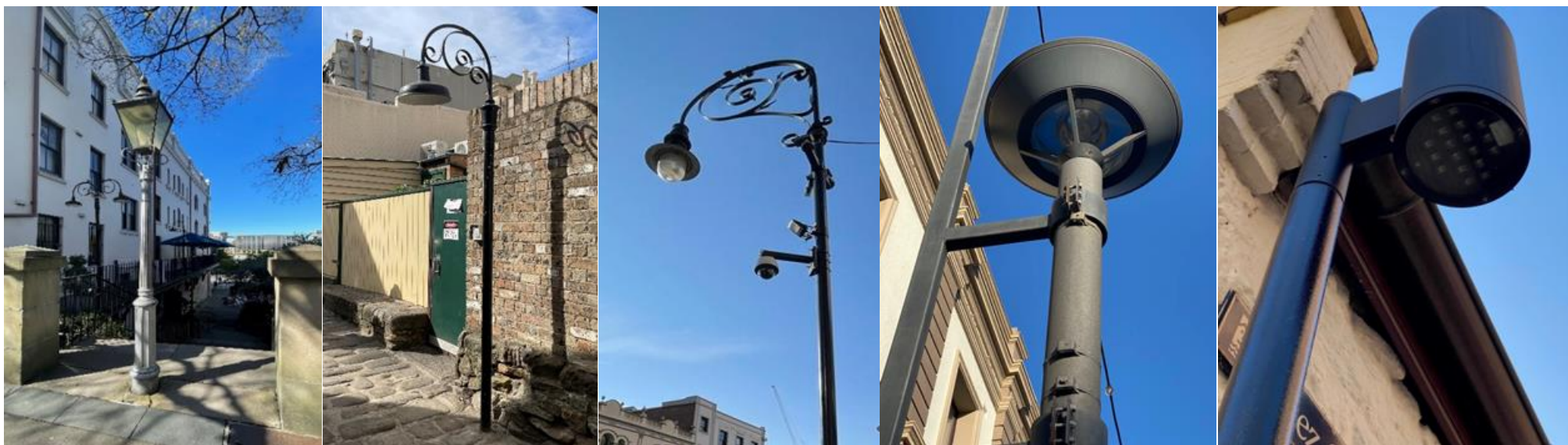
Figure 3.8 Selection of existing streetlights
