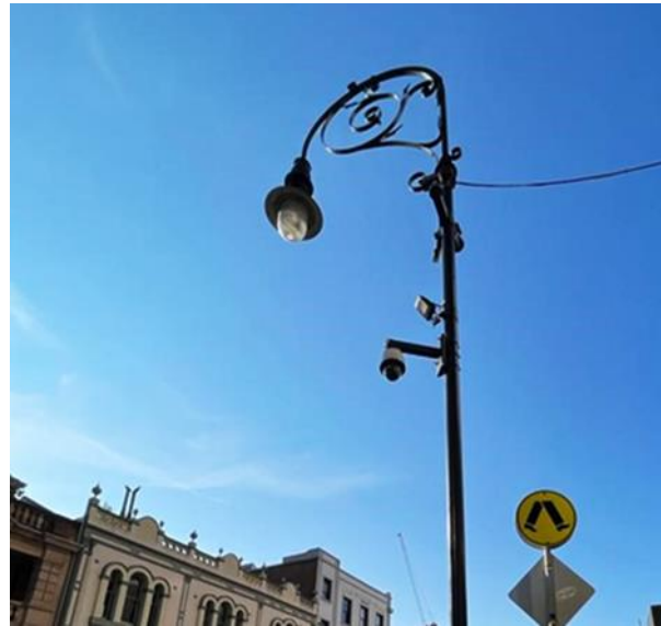
Figure 7.49 Existing heritage poles street poles for retention
