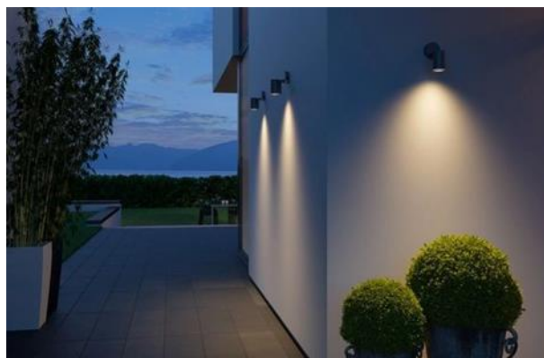
Figure 5.12 Examples of wall-mounted lighting, Ilya Melikhov - Simon Callagan - Steinel
