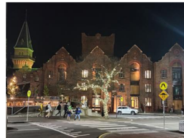
Figure 7.107 Existing crossing at George Street
