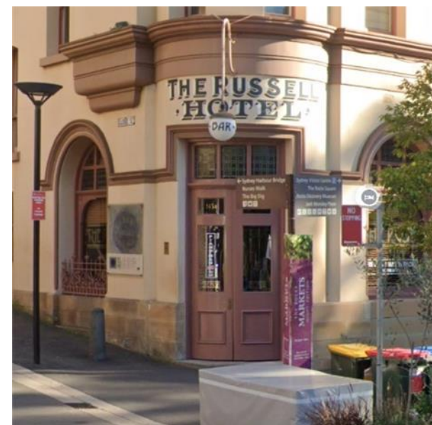
Figure 7.146 Existing round light fitting at The Russell Hotel, George Street
