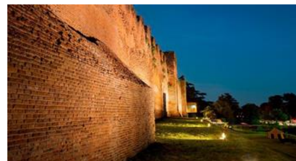
Figure 6.6 Examples of accent luminaires, iGuzzini - Simon Callagan - Linea Lighting
