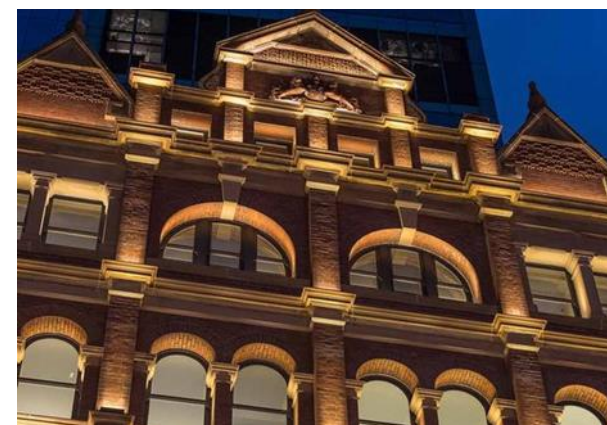
Figure 7.147 Accent lighting highlighting architectural features and grazing the surface of the brick and stone façade, DPA Lighting
